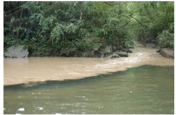
On ALDOT’s watch: muddy water from erosion at a Corridor X road construction site hits Village Creek. Photo by Nelson Brooke.
