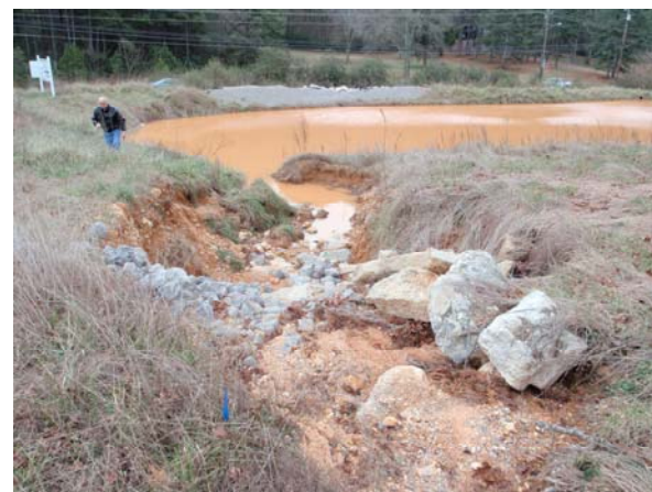
Poor erosion controls allow muddy runoff to fill this sediment pond in Clay. Photo by Nelson Brooke.
