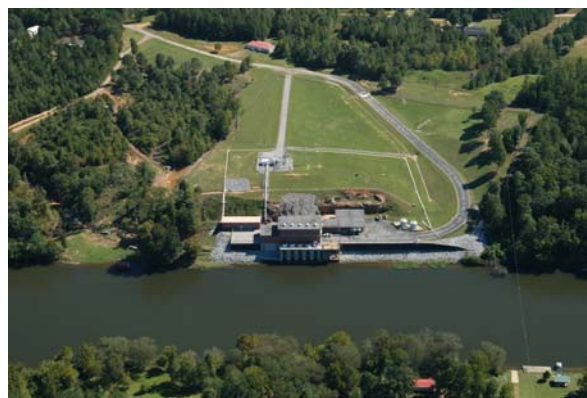
Umicore's significant bromide discharges compromise drinking water from the Birmingham Water Work's Mulberry Fork intake. © Nelson Brooke
