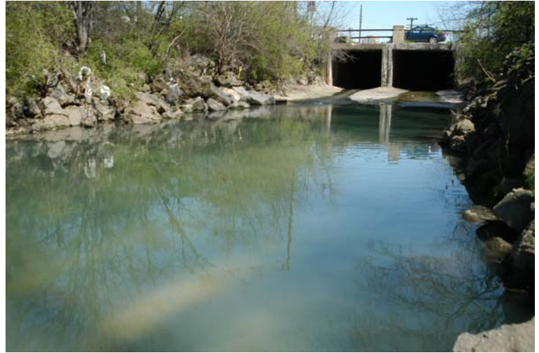
Sewage from an unidentified source enters Valley Creek from these storm sewer culverts at 5th Ave. N & 7th St. N, making the water cloudy. Photo by Nelson Brooke.
