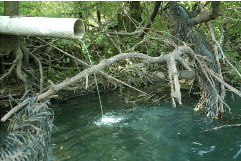
Polluted water far above Birmingham Hide & Tallow's permit limits being discharged into Valley Creek. Photo by Nelson Brooke.
