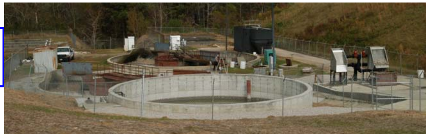
Following Black Warrior Riverkeeper's notice to file suit for 1,060 CWA violations , a new 100,000 gallon surge basin (foreground) was installed at Donaldson WWTP. © Nelson Brooke (November 15, 2005)
