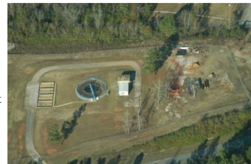
Cordova Wastewater Treatment Plant 518 CWA Violations © Nelson Brooke (Nov. 29, 2005)
