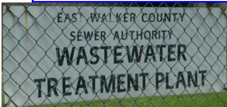
East Walker County Wastewater Treatment Plant 4,473 CWA Violations © Nelson Brooke 2005
