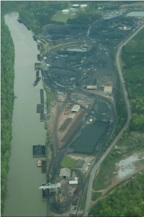
Birmingham is a barge loading facility on the banks of the Locust Fork of the Black Warrior River. This port is Birmingham’s gateway to Mobile Bay, providing for the transport of coal, asphalt, chemicals, wood chips, and steel. © Nelson Brooke Flight provided by SouthWings.org
