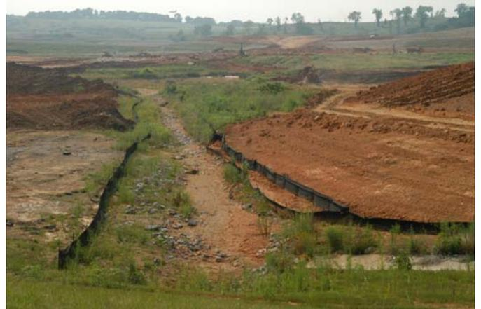
*Prior to site upgrades, inadequate erosion control allowed large amounts of sediment into drainages. Photo by Nelson Brooke.*
