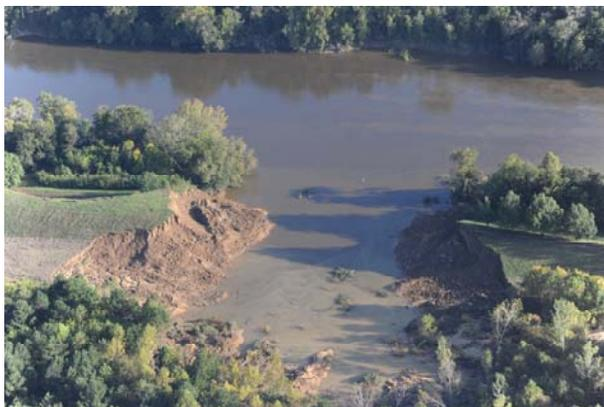
Aerial picture of the US Army Corps of Engineers' dredge disposal dike collapse at Snow's Bend on the Black Warrior River (downstream of Tuscaloosa near Snow's Bend Farm). The Corps of Engineers' Tuscaloosa office estimated that between 300,000 - 500,000 cubic yards of sediment from this multi-acre dike were lost into the river and washed downstream.
