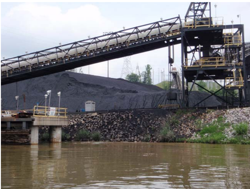
Loose coal falls down the Mulberry Fork's riverbank (dark sections) at the loading dock of Alabama Power's Gorgas Steam Plant. Photo by Nelson Brooke.
