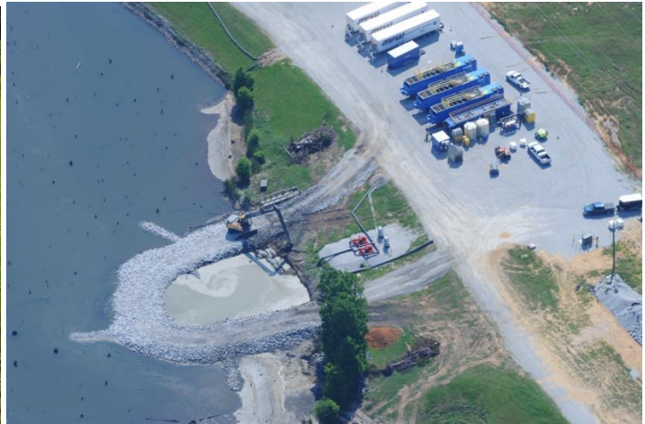
Wastewater pumping and treatment plant for dewatering ash pond
