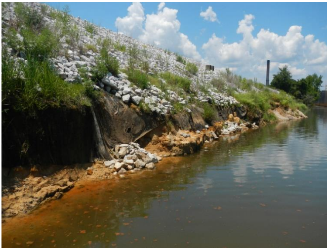
July 2016 | Orange seeps contaminated with coal ash flowing from ash pond dike along eastern barge canal
