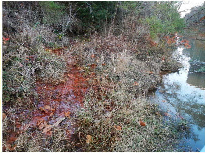
May 2014 | Orange/red seeps contaminated with coal ash flowing from ash pond dike along eastern barge canal | Dec. 14
