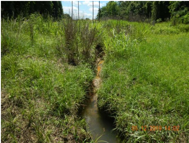
May 2019 | Seep flowing from South ash pond dike
