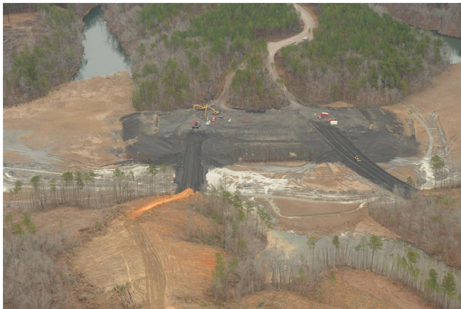
Black material placed in Rattlesnake Lake and ongoing road construction.
