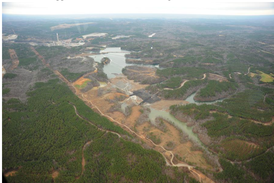
Rattlesnake Lake coal ash impoundment. Headwaters of Rattlesnake Creek in foreground.
