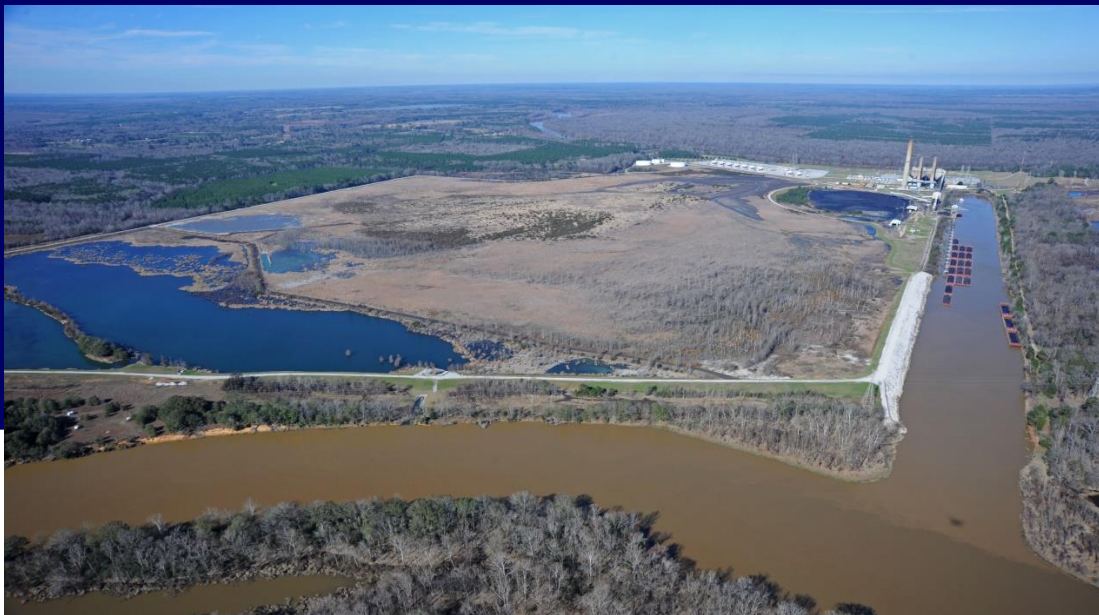
Plant Greene County Ash Pond (middle), Black Warrior River (foreground) | Flight by SouthWings.org
